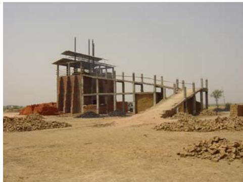
The unique feature in this VSBK is the construction of an elaborate L-shaped RCC ramp. This is not only used for green brick transportation to the loading platform but also as a store area for green bricks to be used for firing during rainy season.
